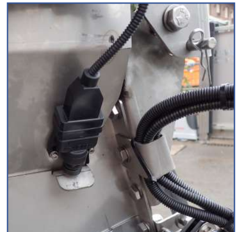
Safety microswitch on the spreading tower
